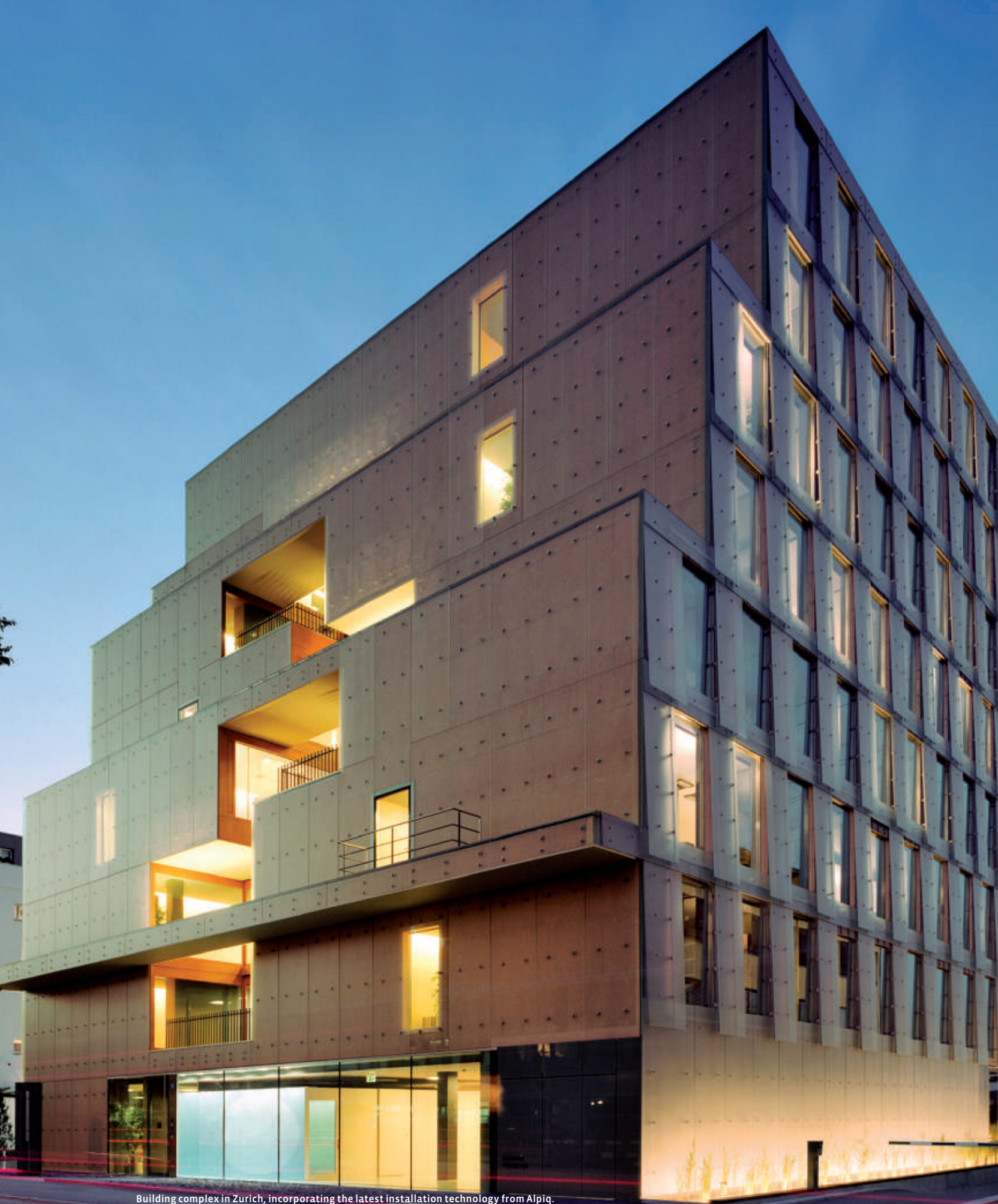
Building complex in Zurich, incorporating the latest installation technology from Alpiq.
